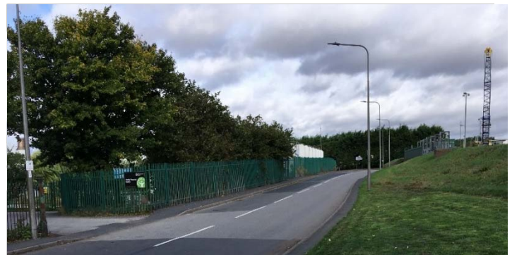
Photo showing front of Keadby Pumping Station location of temporary traffic lights
